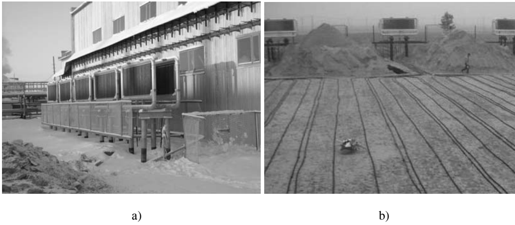
FIG. 10: Cooling systems: a) condensers; b) laying of horizontal cooling profile
