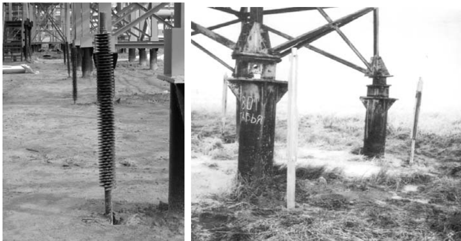
FIG. 5: Seasonal cooling devices with one vertical condenser
