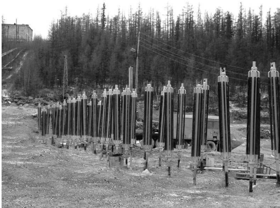
FIG. 11: Application of subsurface seasonal cooling devices for creating cutoff curtains
