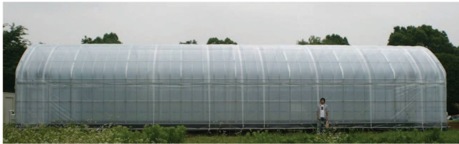
FIG. 4: Greenhouse used in mist cooling testing.
