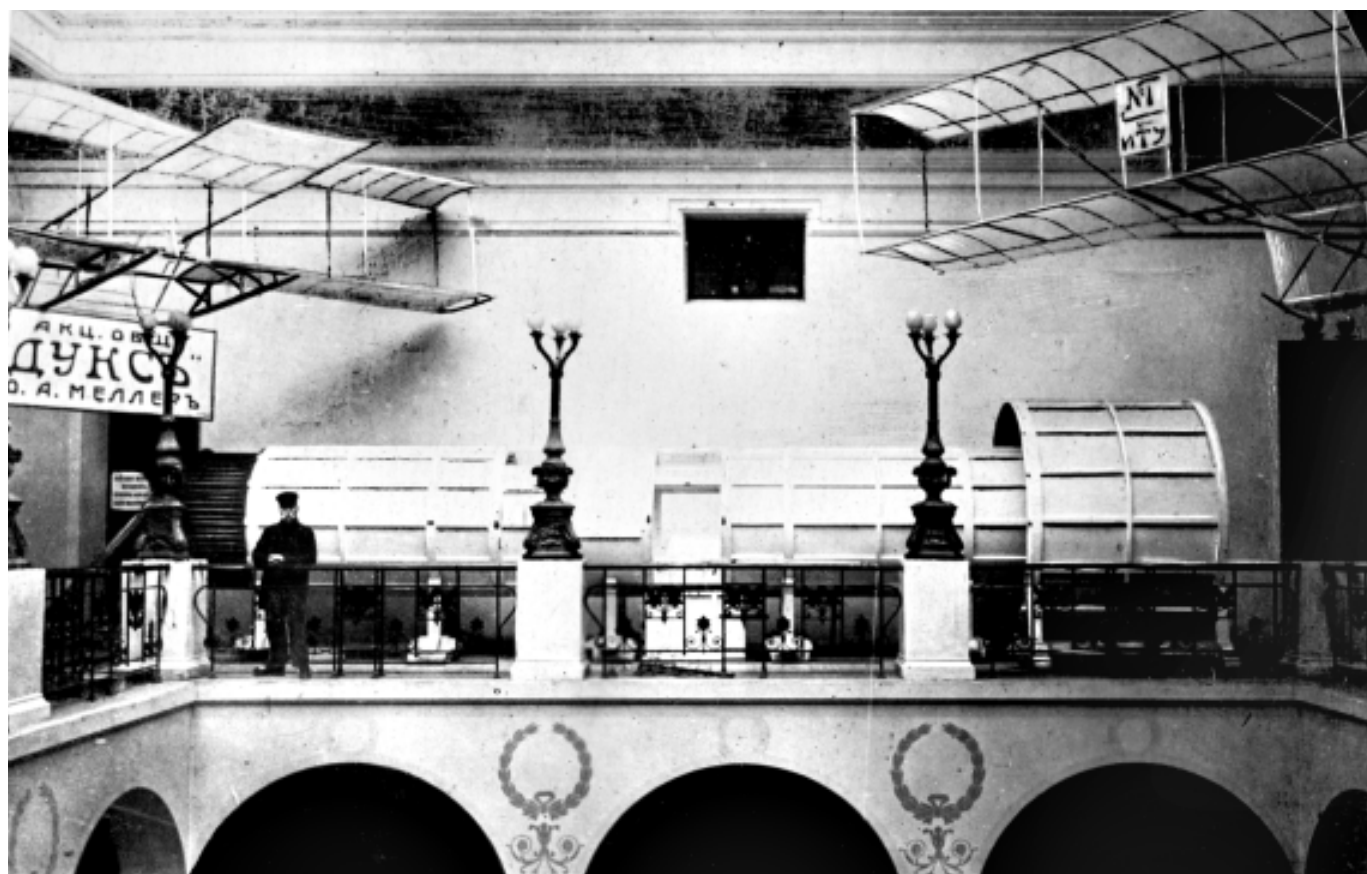
Aerodynamic tunnel built in MSU (Moscow State University) at the initiative of N.E. Zhukovsky
